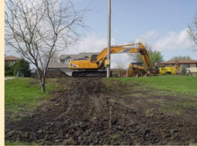
Construction equipment has run over the root zone of the tree.
